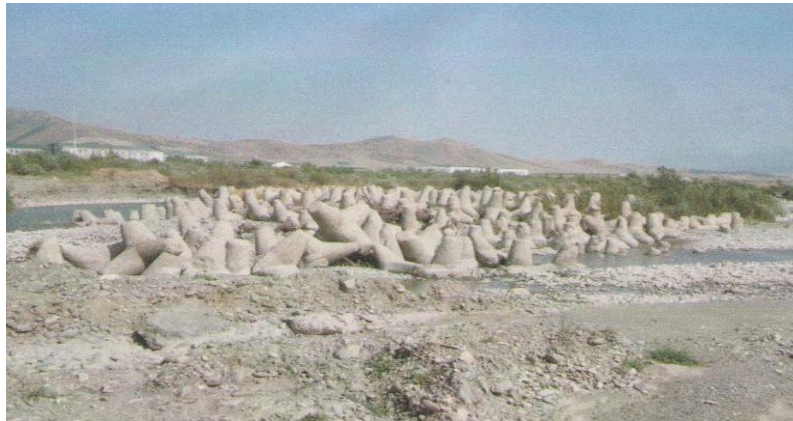
Fig. 2. Tetrapods at the bridge on the Liakhvi River, Georgia [15]
