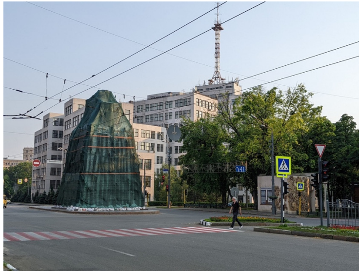
Fig. 11. The Derzhprom House from the side of Nauki Avenue at the beginning of the war. Kharkiv, 11.07.2022
