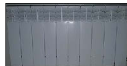
Fot. 1. Aluminiowy grzejnik c.o. Photo 1. Aluminium central heating radiator
